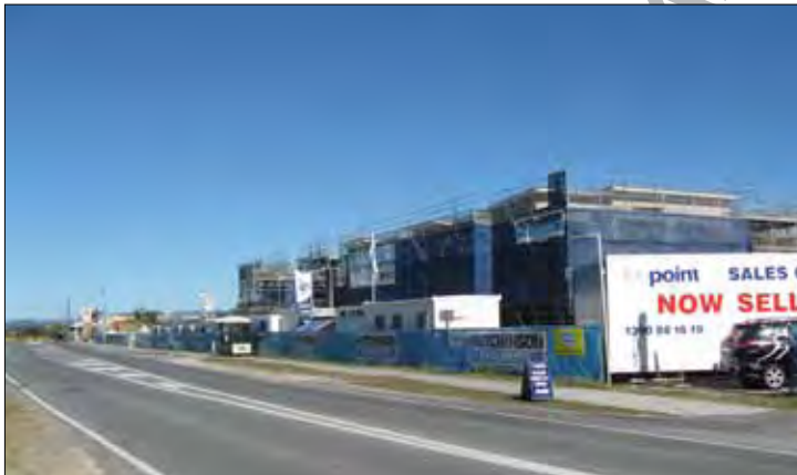
The Point - under construction
