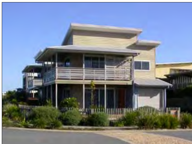
From the Tweed Coast Road buildings are designed to appear as single residential dwellings although a lot may contain more than one dwelling. Building length along the road is similar to a large house, landscaped setbacks and front doors and windows to the road provide a residential and coastal quality.
