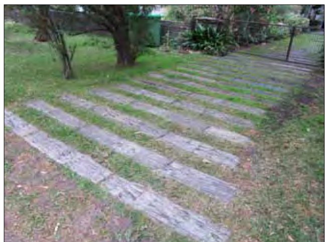
Alternative solutions to concrete and bitumen hard stand areas are to be used on both new and existing lots.
