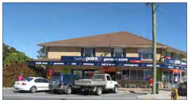
Existing retail building
