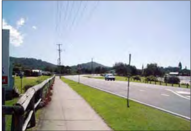
Existing view Looking North along the Tweed Coast Road
