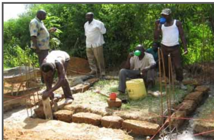
Starting the construction of the kiosk
