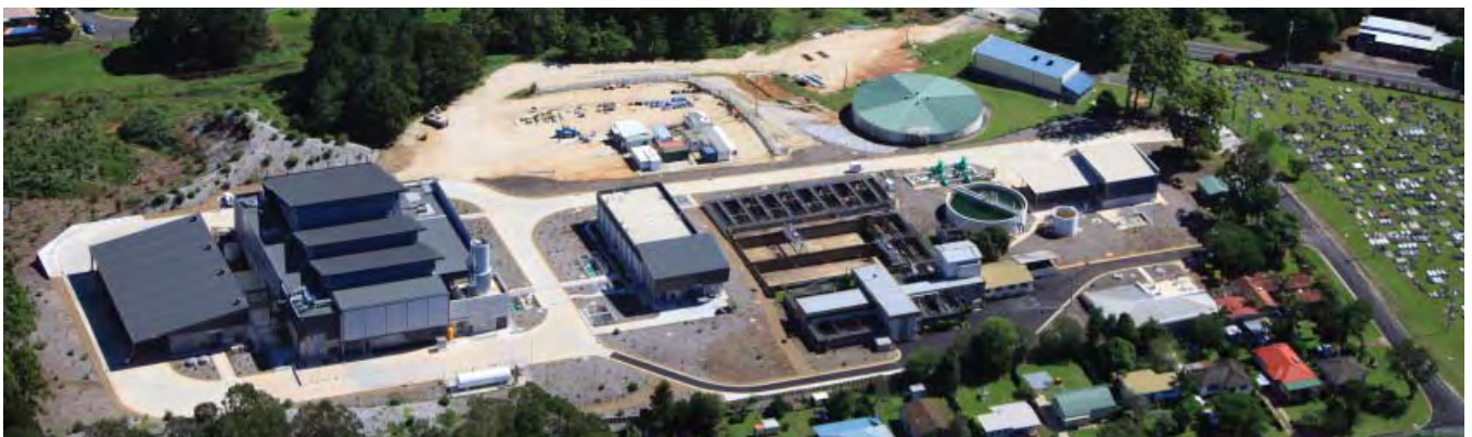
Bray Park Water Treatment Plant
