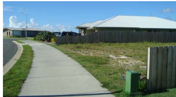
Photograph 4 – Site frontage, looking north Source: CPS – February 2010
