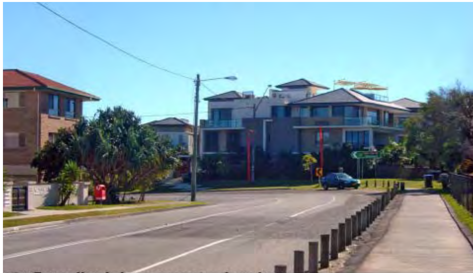
Compliant temporary structure 1:1.3
