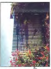
1500h aluminum permeable fence and gates to Casuarina Way - Lots 7 - 13 Refer Sheet 01/18
