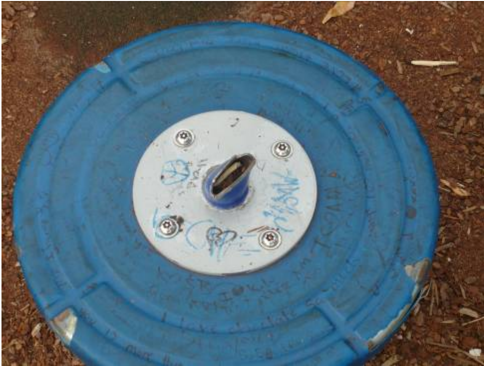
Figure 3: The spinner in figure 1 had the safety scrim removed/stolen and the remaining pole snapped off prior to being replaced.
