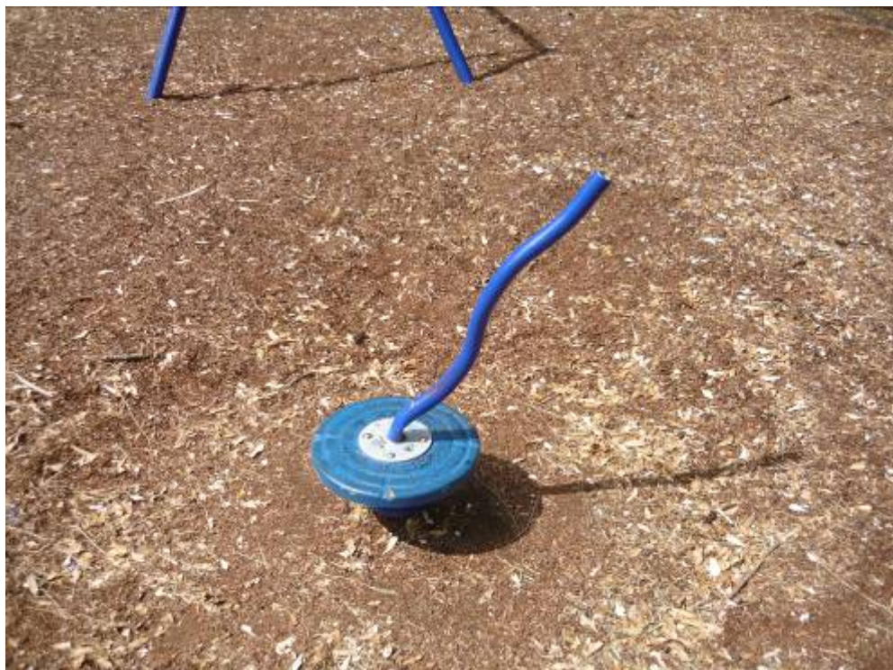
Figure 2: The 'spinner' was broken and bent. Safety scrim was erected and a replacement spinner ordered.
