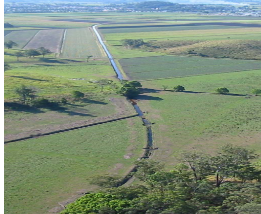
Blacks Drain. Acid Sulfate Soil research site An University of NSW and Tweed Shire Council ARC Linkage Project
