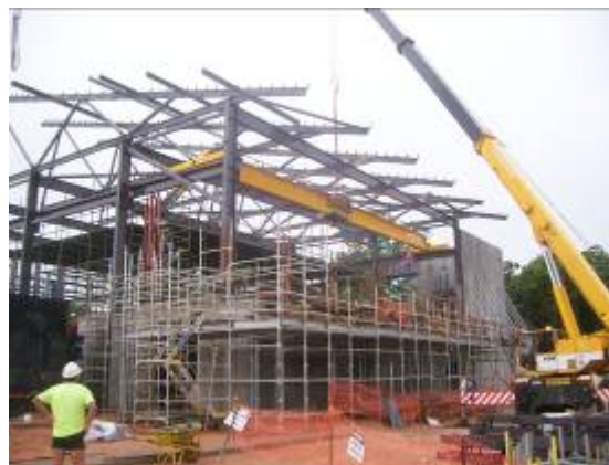
Construction at the Bray Park Water Treatment Plant
