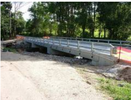
Replacement of timber bridge
