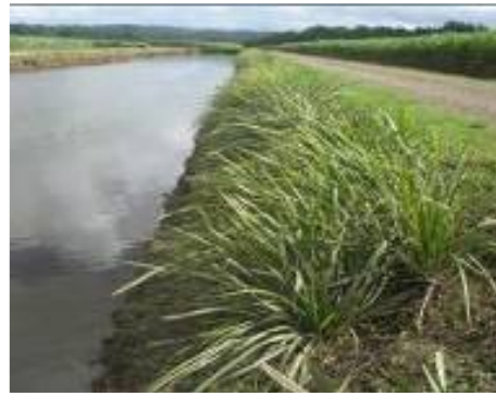
Vegetative buffer strips controlling drain bank erosion and farm runoff
