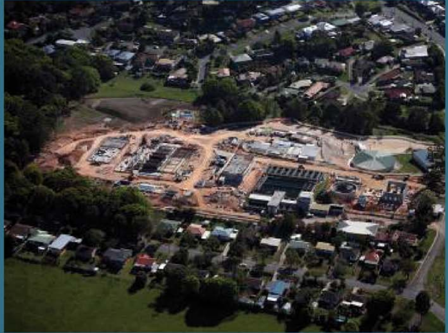
Bray Park Water Treatment Plant construction site
