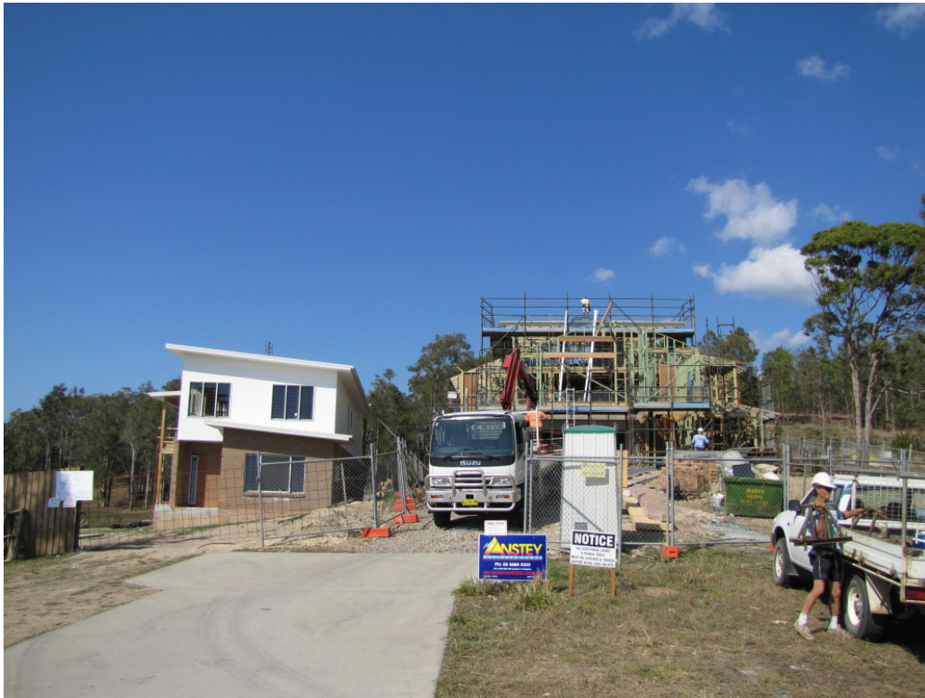
Photo 1 (above) depicts the subject property (which is seeking approval for an increased height limit of 125mm for the constructed home) on the left and the objector's home (which is also under construction) on the right.
