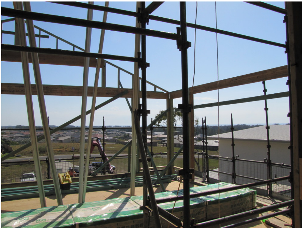
Photo 4 (above) is taken from the objector's home presently under construction and indicates that to the north there is an extensive outlook available.
