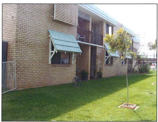
view from Tupia looking east towards Banks Avenue.
