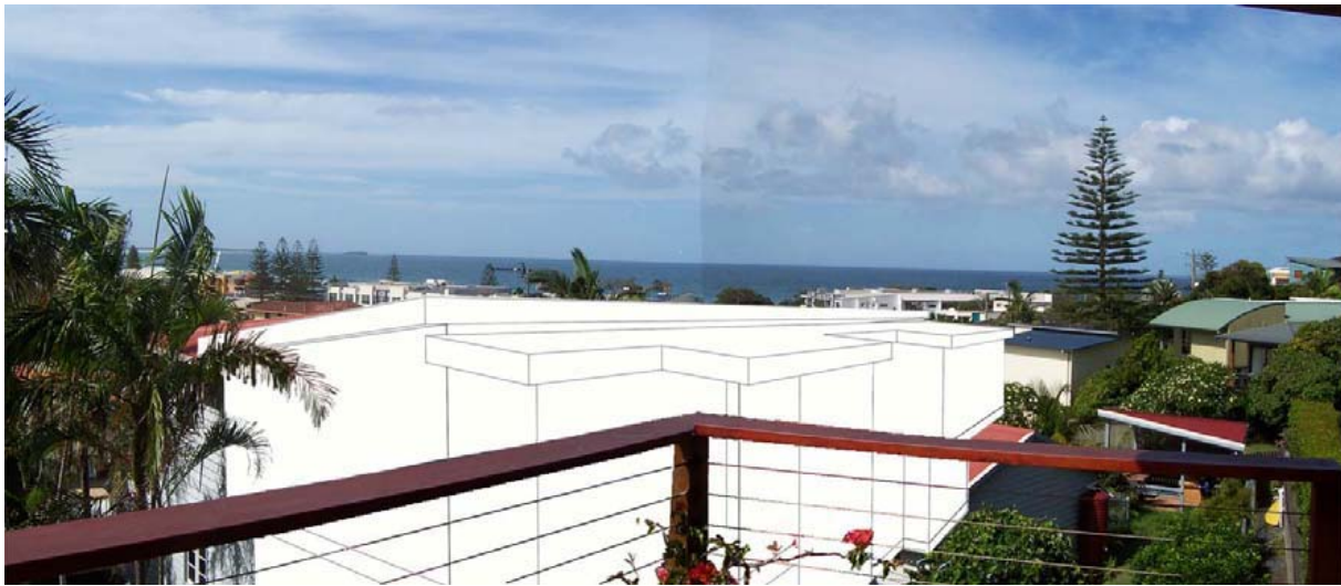
Figure 9- Solid overlay view north from 5 Rob Roy Crescent main outdoor balcony
