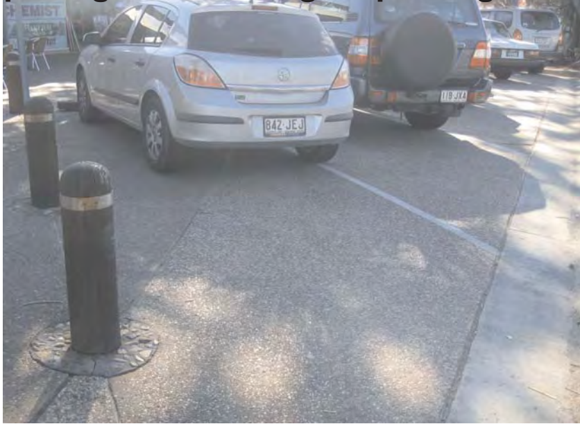
paving finish to angled parking
