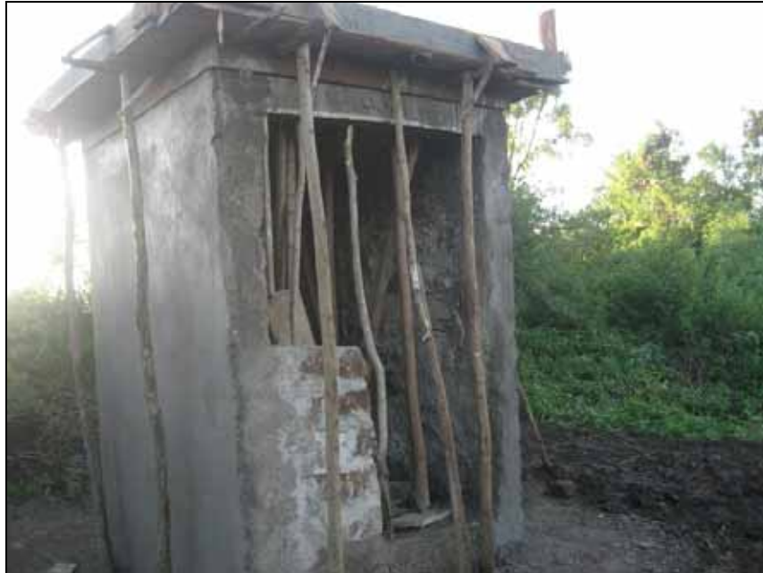
A small but incredibly challenging project – the water kiosk...not quite finished.
