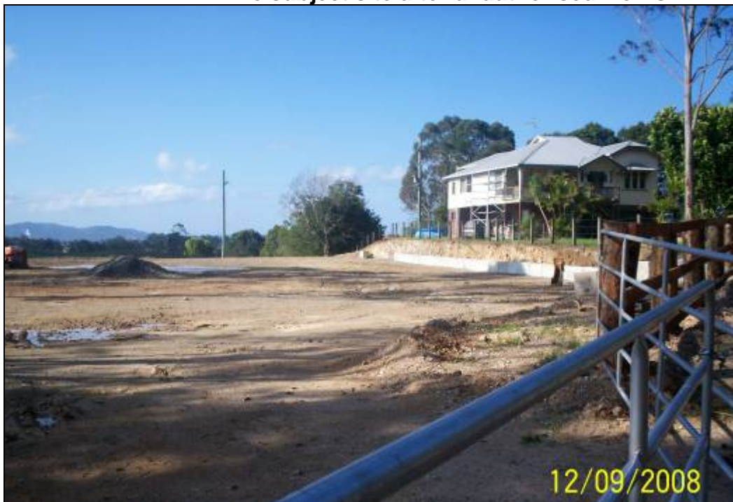
The subject site after unauthorised works
