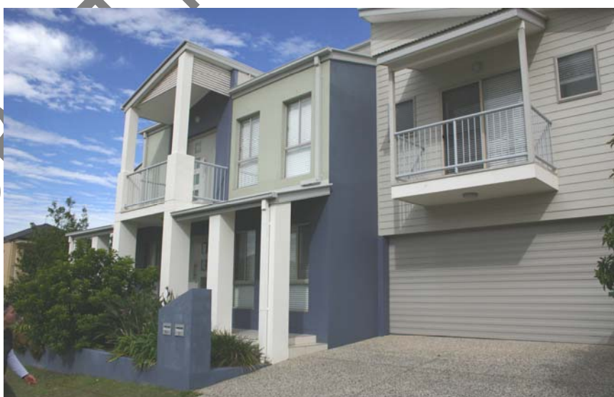
The visual impact of this garage has been reduced by making the garage door a similar material and colour to the wall so the garage reads as the wall to the building, it is also set back from the main façade of the building.
