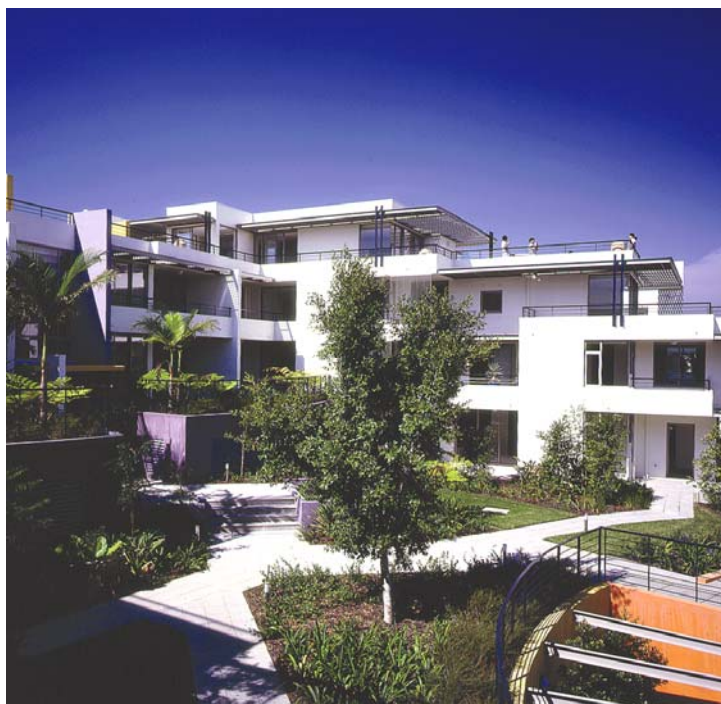
Communal open space areas can provide a pleasant outlook for dwellings and shared facilities such as pools and gardens.
