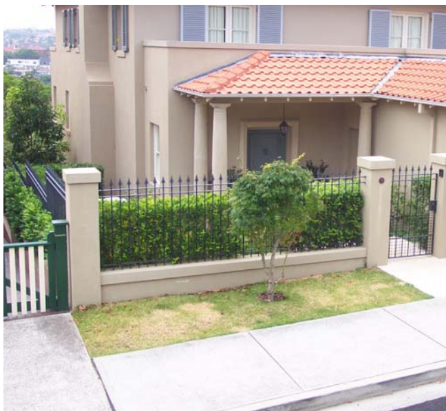
This fence returns down the side boundary, combines landscaping, open fencing and low walls to create a fence that enhances the pedestrian scale and residential qualities of the street.
