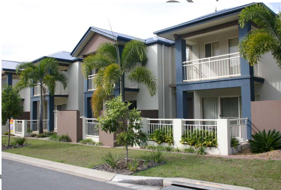
These Row Houses have been designed to orient to and address the street by having habitable rooms facing the street.
