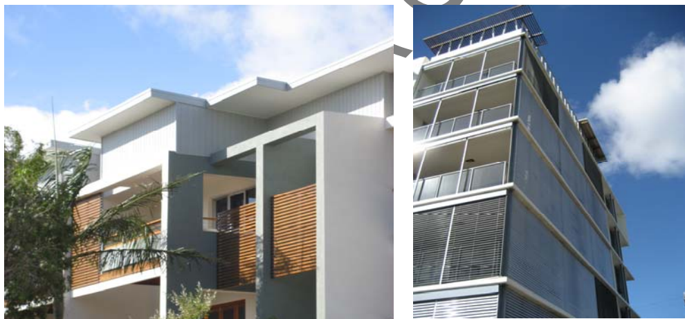
Operable and moveable louvers allow the amount of visual privacy, outlook and sun penetration to be controlled by the residents to suit different personal requirements and times of the day or night.
