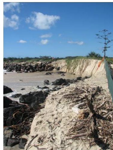
Coastal erosion at Duranbah Beach following a series of harsh weather events in February 2008
