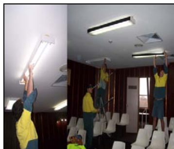
Energy efficient lighting being installed in the Council Chambers
