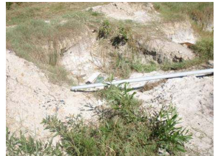
Picture. 6 - Uneven ground within beach foredune areas.
