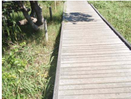
Picture. 5 – Kick rails provided on paths in vicinity to Norries Head lookout.
