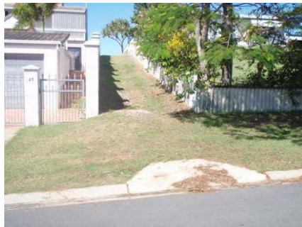
Picture. 5 – Defined access path in residential zone with any hazard signage.
