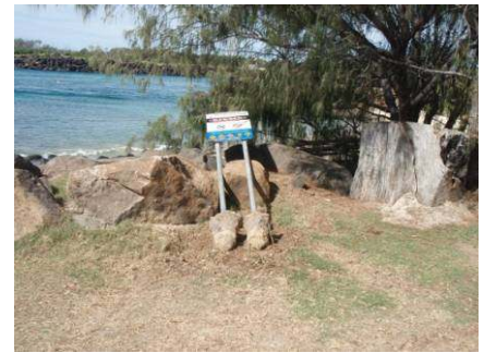
Picture. 6 - Removal of hazard signage noted at time of assessment.
