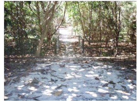
Picture. 3 – Defined access with no hazard signage.
