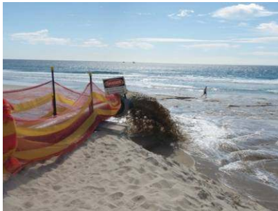
Picture. 4 – Sand pumping delivery point onto Duranbah Beach. No preventative/ distance barriers noted at time of assessment.
