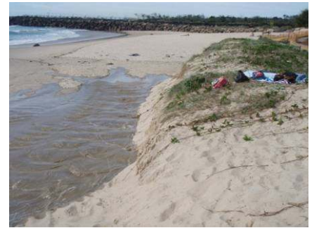
Picture. 3 – Drop off on Duranbah beach due to eroding sand dunes.
