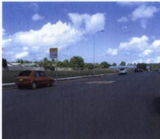
Corporation Circuit Site
