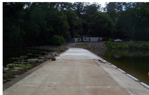
A complete refurbishment of the Bray Park weir occurred in 2006. The crest steel grillage of the weir used to contain the rock fill embankment was removed and replaced with a structural concrete cap at a project cost of $2.2(M). Water to the Bray Park treatment plant is drawn from the Bray Park weir.
