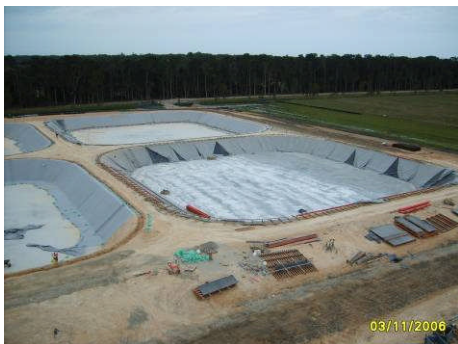
Construction of main processing tanks at the new Kingscliff sewerage treatment plant site
