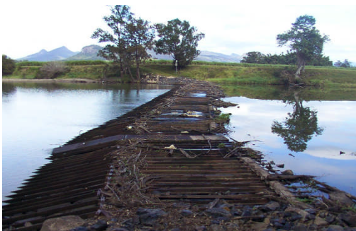
A complete refurbishment of the Bray Park weir occurred in 2006. The crest steel grillage of the weir used to contain the rock fill embankment was removed and replaced with a structural concrete cap at a project cost of $2.2(M). Water to the Bray Park treatment plant is drawn from the Bray Park weir.
