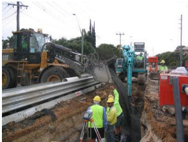
Kennedy Drive works 2006
