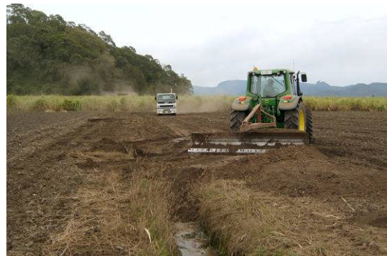
Filling of excess drains to reduce the export of acidity from acid sulfate soils
