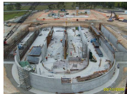
Construction of main processing tanks at the new Kingscliff sewerage treatment plant site
