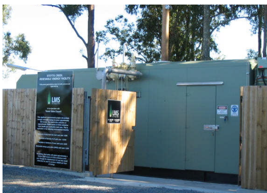
Landfill gas management at Stotts Island. The methane gas extraction system feeds electricity into the power grid
