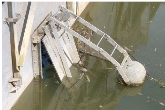
A floating arm opens the floodgate and allows water exchange with each tide. The gate opens on the low tide and closes with the rising tide to improve fish passage and habitat and water quality
