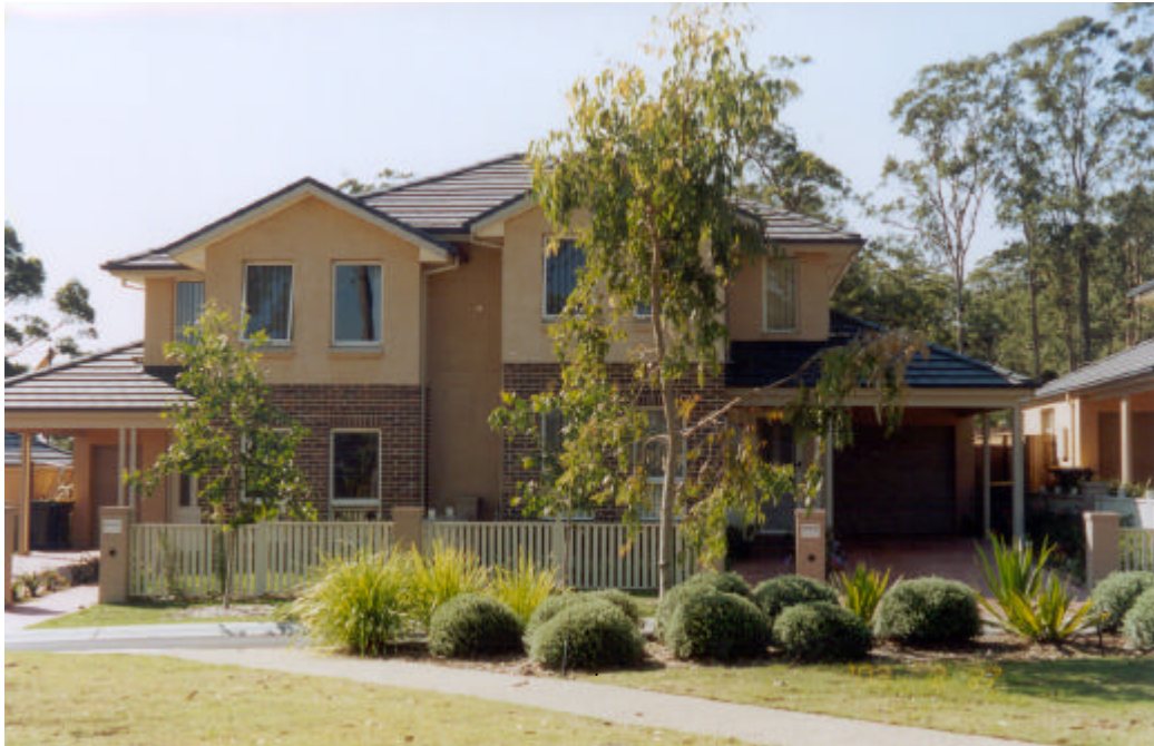
Dual Occupancy Housing has its carparking set well back from the buildings front elevation so as not to dominate the streetscape.
