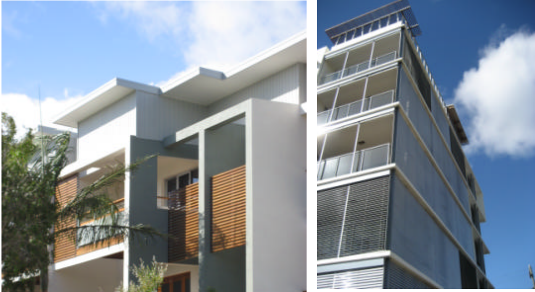
Operable and moveable louvers allow the amount of visual privacy, outlook and sun penetration to be controlled by the residents to suit different personal requirements and times of the day or night.
