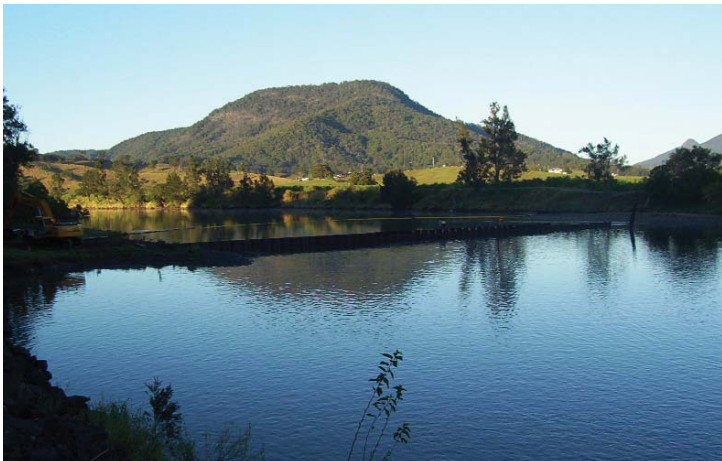
Bray Park Weir
