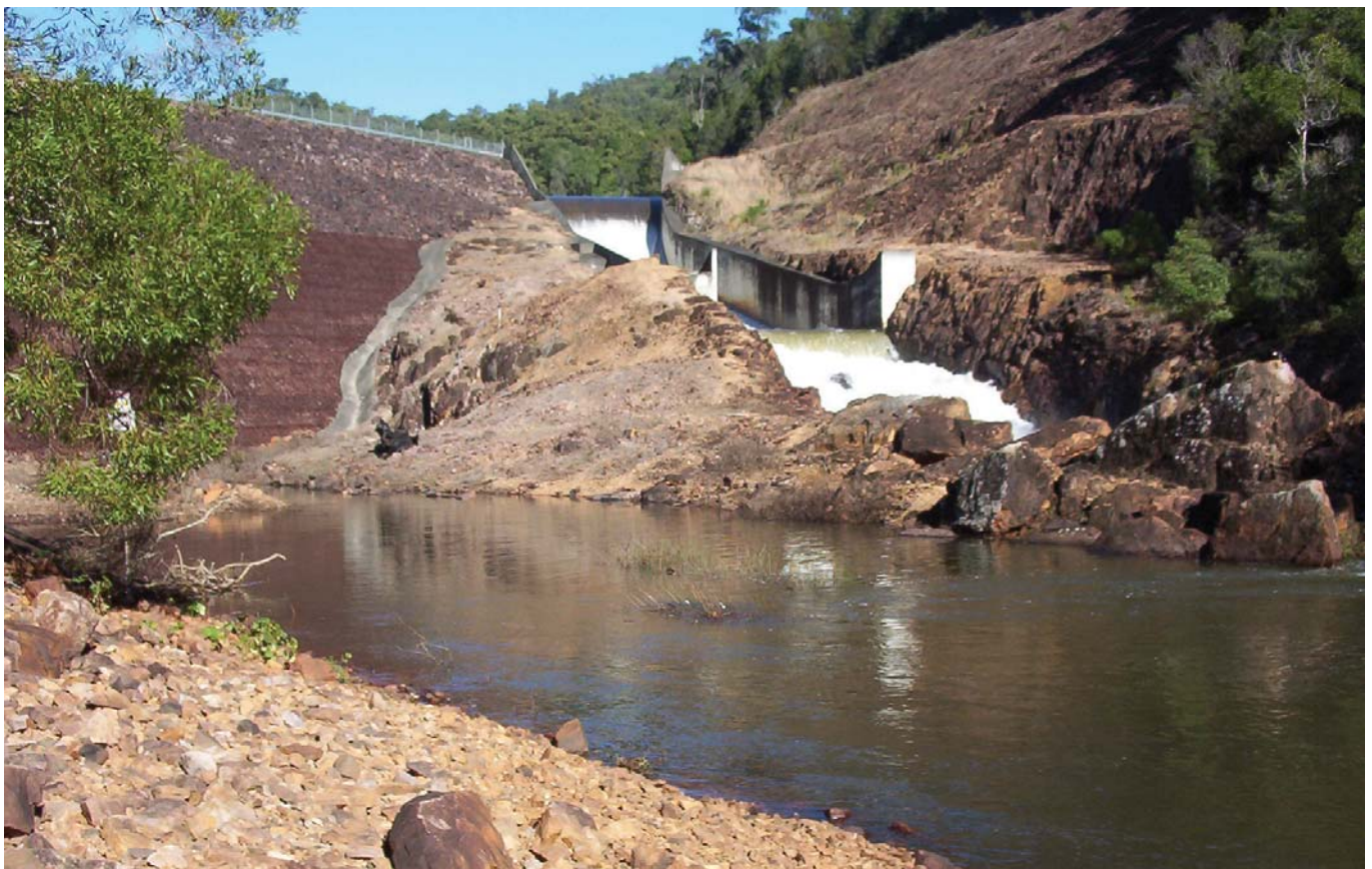
Clarrie Hall Dam
