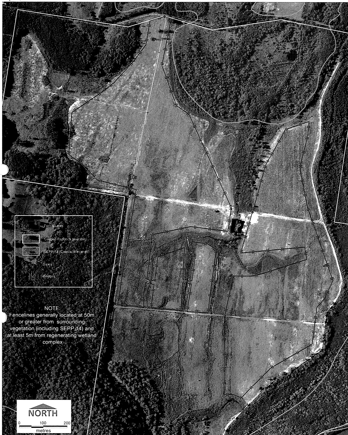
Figure 1 - Aerial Photograph as per Condition 2
