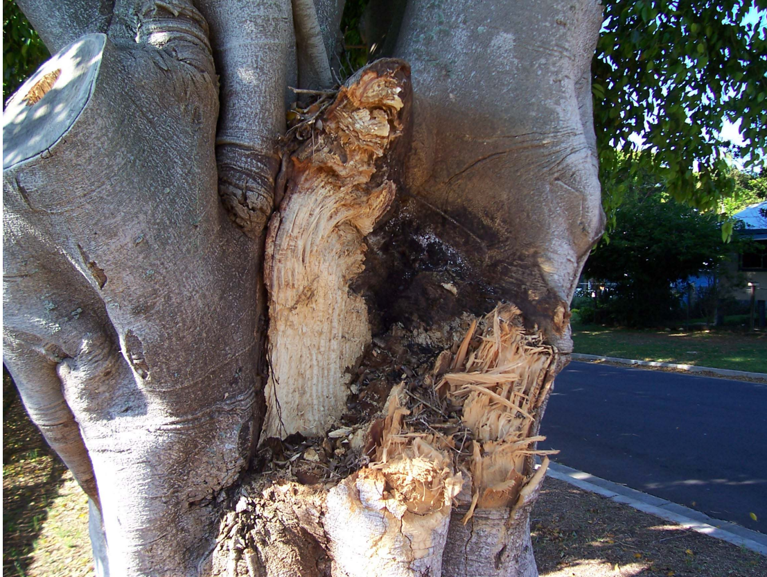
Figure 3 Wound in fig tree Crescent Street as result of limb drop, 23 November showing evidence of decay
