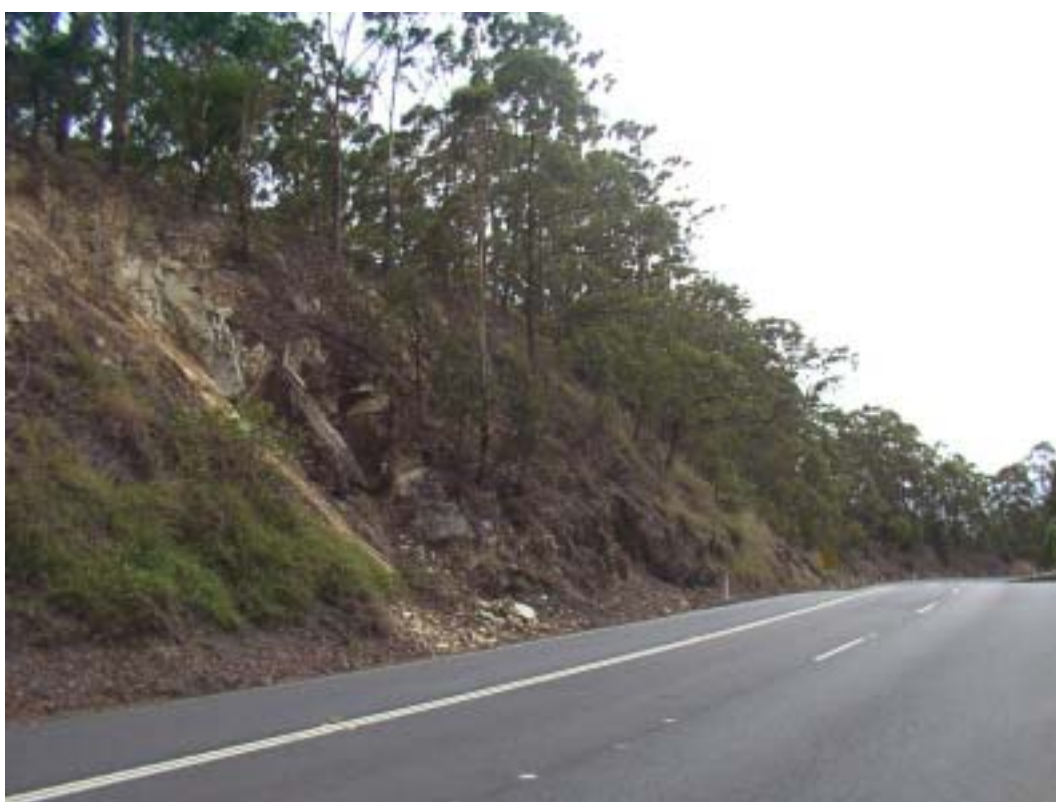
Photograph 2. Overhanging rock section at distance 60m
