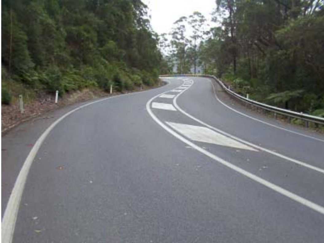
Photograph 3. Example of proposed linemarking to keep opposing traffic separated south of the slope
