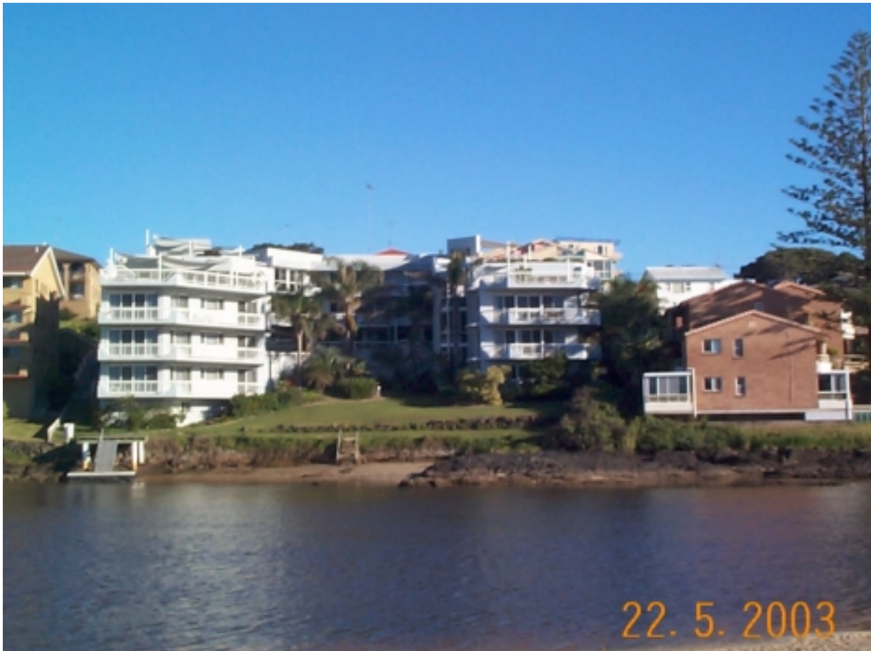
FIGURE 2 – EXISTING BUILDING VIEWED FROM OPPOSITE SIDE OF CUDGEN CREEK
