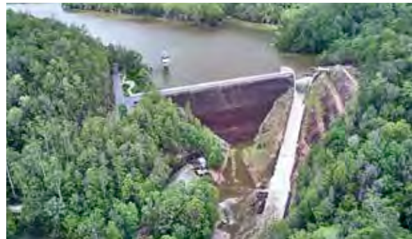
Clarrie Hall Dam.
