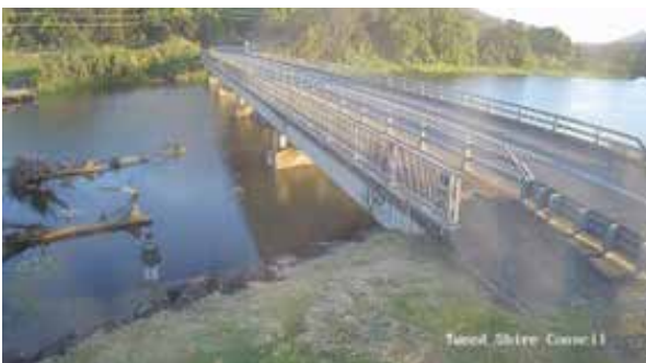
An image from the flood monitoring camera at Byangum Bridge.
