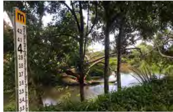
The new flood gauge at Crabbes Creek.
