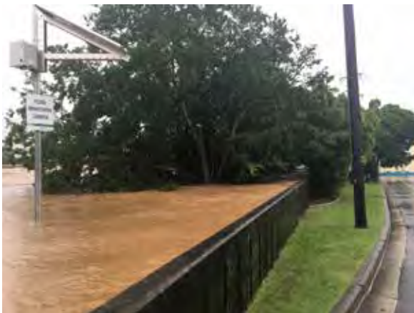
Holding back the waters: Murwillumbah CBD levee at Wharf Street just after 5 pm on 28 February 2022.
