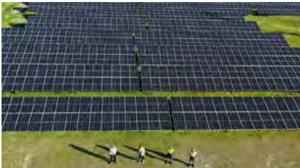
Caption: Tweed Shire Council staff stand proud in front of the Tweed's biggest solar array, housed at the Banora Point Wastewater Treatment Plant.
