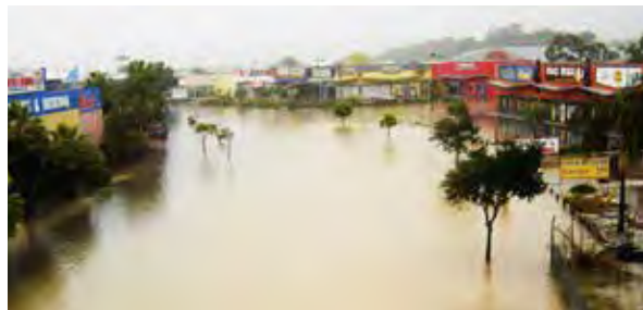
Flooding on Greenway Drive, Tweed Heads South in 2005.
