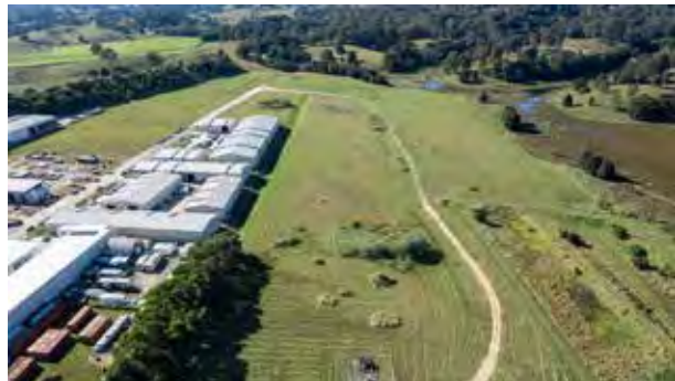
The Industry Central Land Swap project is a strategic solution to assist selected businesses located within the high flood risk zone in the existing South Murwillumbah industrial estate to relocate to flood free land at Lundberg Drive (Industry Central) via a land swap agreement.
