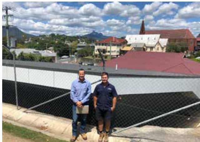
Council's Project Manager – Contracts Daniel Boyle and Jackson Hardy from Hardy Electrical and Solar carry out a pre-inspection for the solar installation at Tweed Regional Museum, Murwillumbah.
