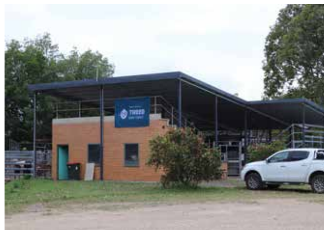
A new brick and steel grandstand replaced the old rotting timber one at Murwillumbah cattle saleyards.
