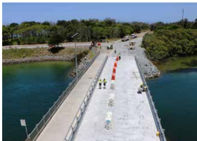
Kingscliff Bridge over Cudgen Creek nearing completion, November 2016.
