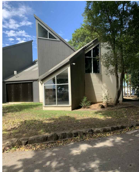
Demolish existing Visitor Information Centre (World Rainforest Centre)
