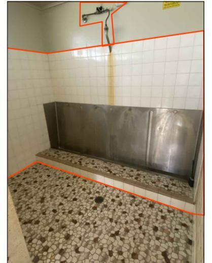
URINAL LOCATED IN MALE TOILET TILES AND PLUMBING SENSOR TROUGH SYSTEM TO BE DEMOLISHED
