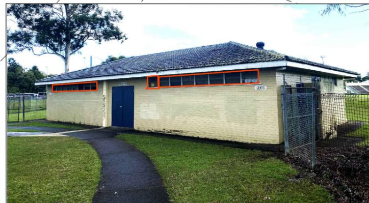
ALL GLASS AND INTERNAL FRAMES IN ENTIRE BUILDING TO BE REMOVED AND DISPOSED WINDOW TIMBER REVEALS TO REMAIN
