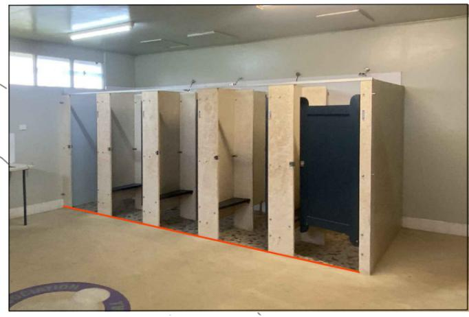
ALL FLOOR TILES IN SHOWERS TO BE GRINDED TO ALLOW EPOXY OVERLAY
