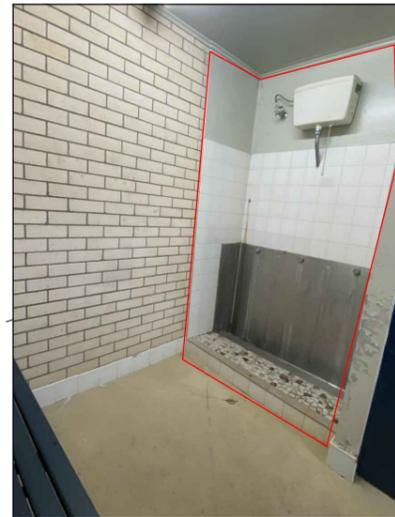
URINALS LOCATED IN CHANGE ROOMS TILES AND PLUMBING SENSOR TROUGH SYSTEM TO BE DEMOLISHED
