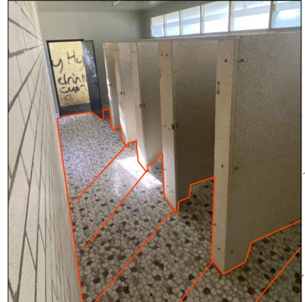
ALL TILED FLOORING TO BE GRINDED TO ALLOW EPOXY OVERLAY
