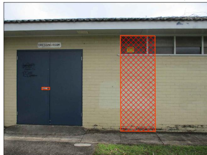
SOUTHERN ENTRY - EXISTING LOCK TO BE REMOVED AND DISPOSED. SAW CUT BRICKS AND PART OF WINDOW REVEAL TO SUIT OPENING FOR 920mm ACCESSIBLE DOOR AND WINDOW FRAME EXTENSION
