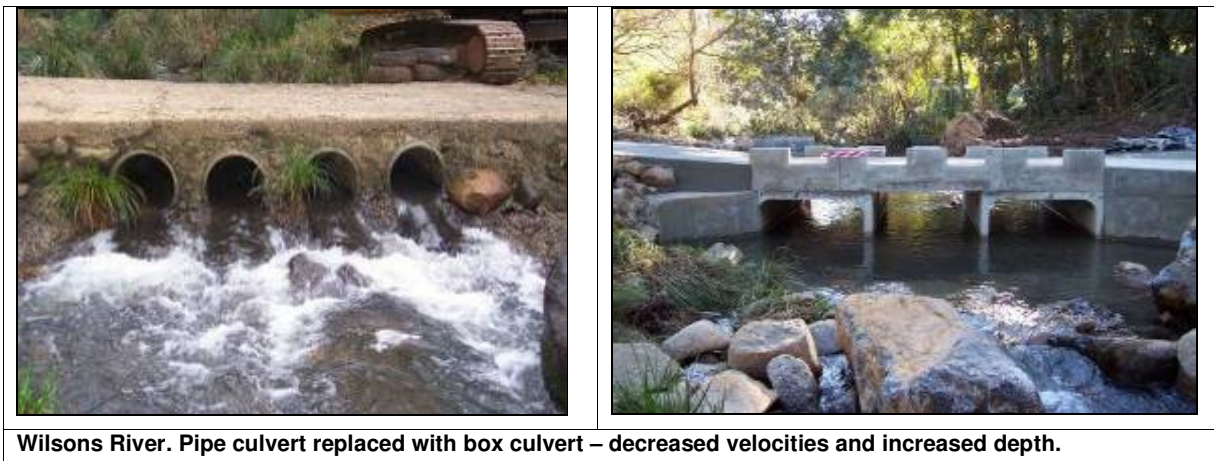
Figure 13.15. Examples of fish passage barriers that have been successfully retrofitted in Northern New South Wales,
