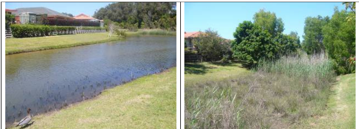
Figure 13.11. Example of parts of the Western Drainage Scheme including a deeper channel with less pollutant removal capacity and higher flood mitigation capacity (left) and shallower, densely vegetated channels providing higher pollutant removal capacity.
